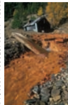
Thousands of abandoned mines on public lands poison streams and groundwater with acid, metal-laced drainage. This old mine in Montana drains into the Blackfoot River, the setting of Norman Maclean's book, A River Runs Through It .
